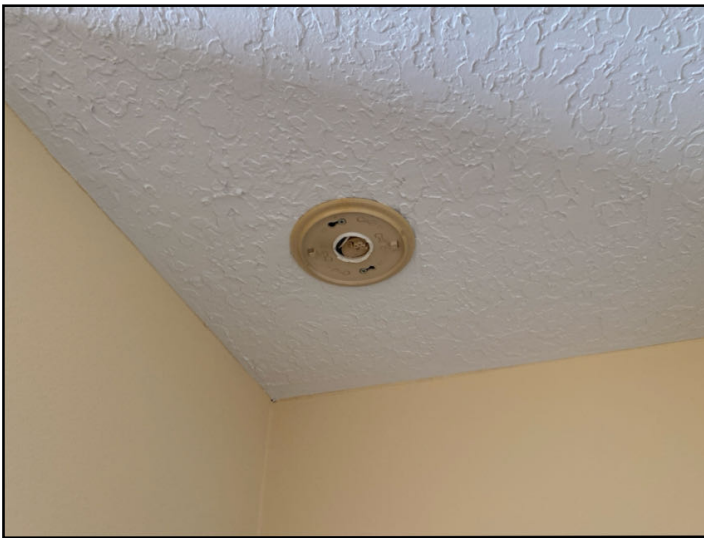
There are a few missing smoke detectors
