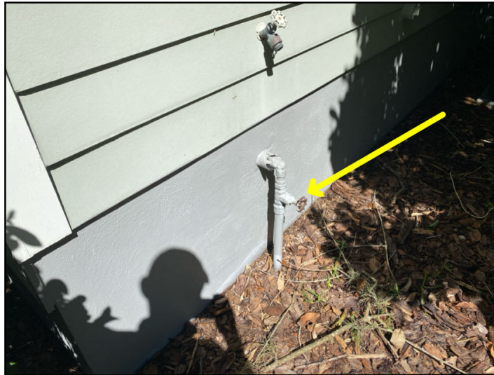
The main water shutoff is on the right side
