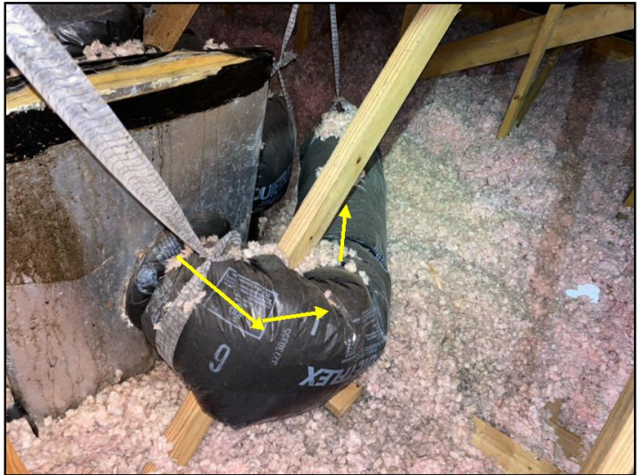
Some ducts have sharp bends. This will reduce airflow to these rooms/vents.
