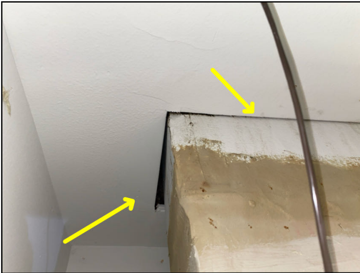
Seal around the duct
