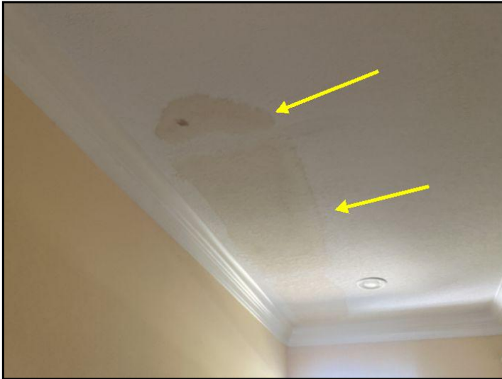
Stains on the ceiling above the front entryway.
