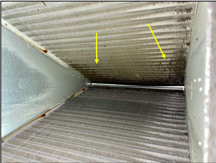
The coils and blower blades are a little dirty and could use a cleaning
