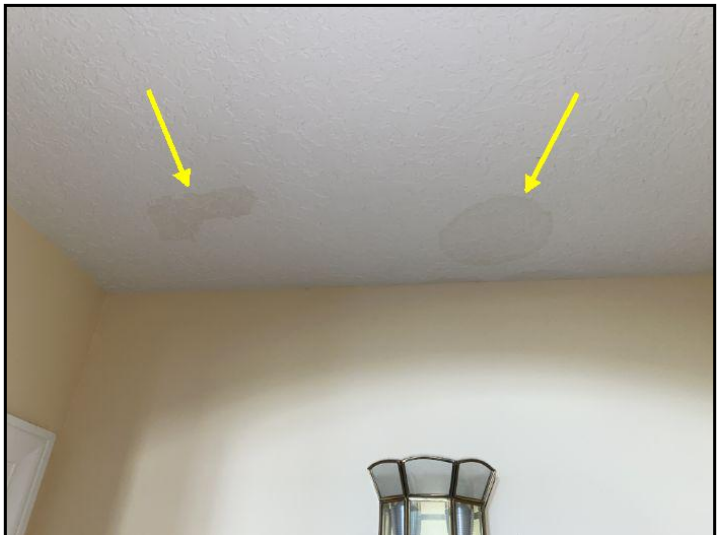
The two spots below the downstairs air handler are dry. This may have been from a past condensate line backup.
