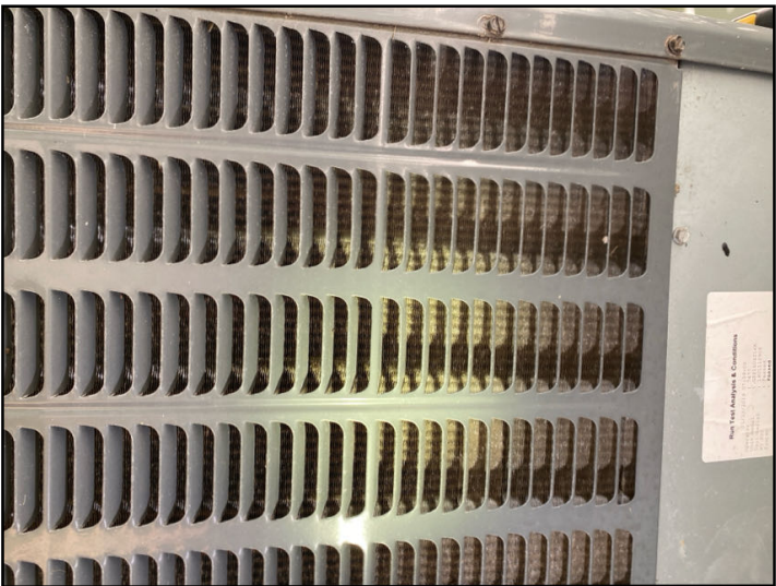
Both units have dirty coils that need to be cleaned
