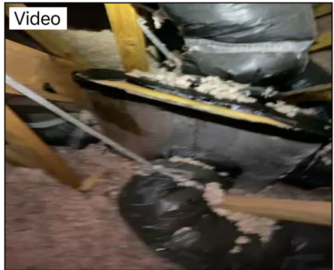
Video showing the air leak
