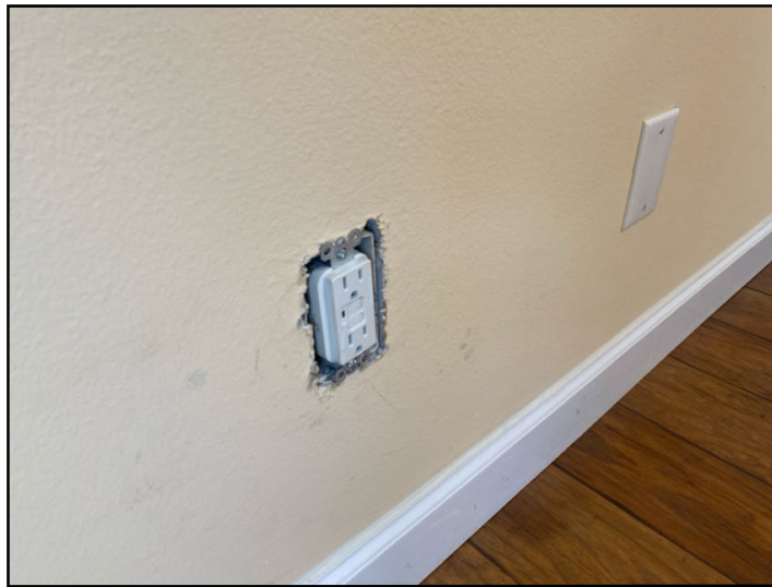
A cover plate is needed for this outlet in bedroom 3
