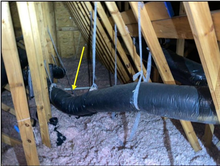
Portions of the ductwork have sags and need to be supported. Sags will reduce airflow
