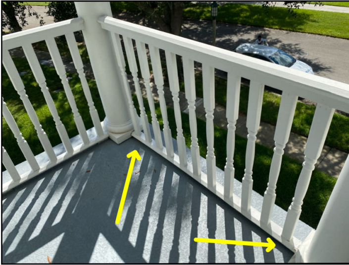
The bottom of this guard rail is not secure.
