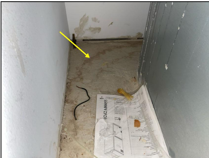
There are stains on the flooring around the downstairs unit from past leaks. The flooring is bowed downwards due to this.
