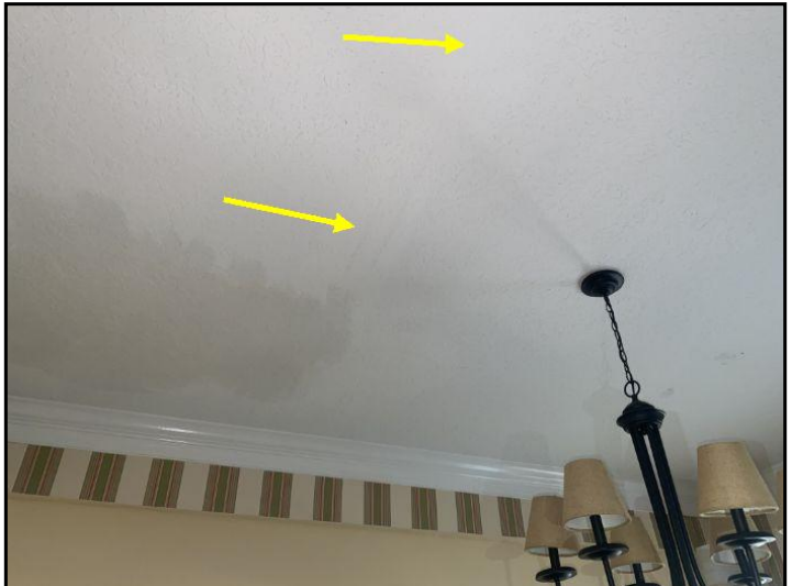
There is a stain on the ceiling in the dining room. The spot was wet when tested today.
